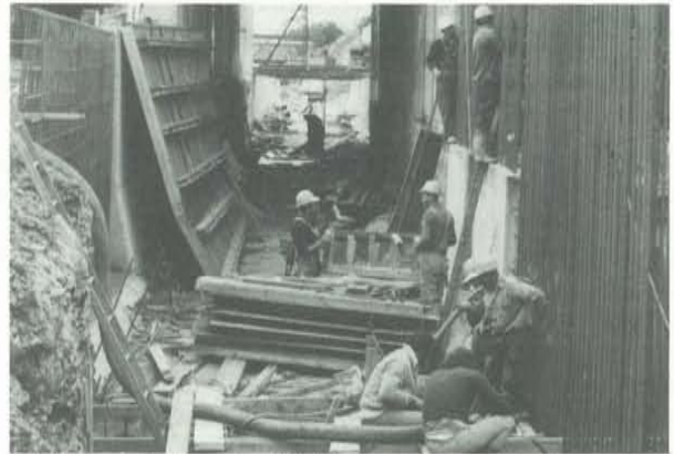
Melbourne Underground Rail Loop — entrance under construction.
