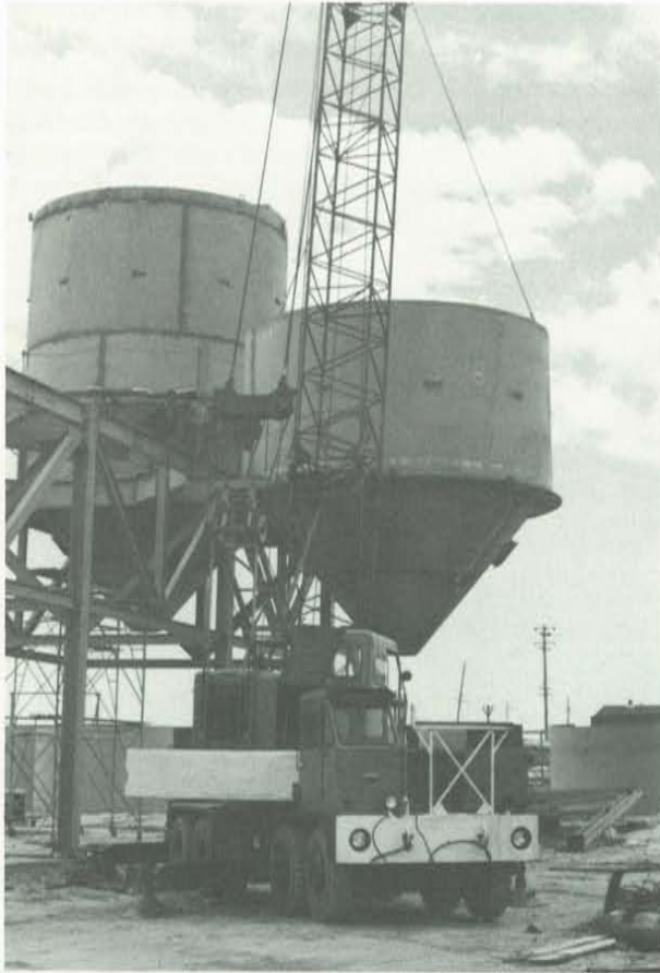
Albion-Reid. Erection of the second bin.
