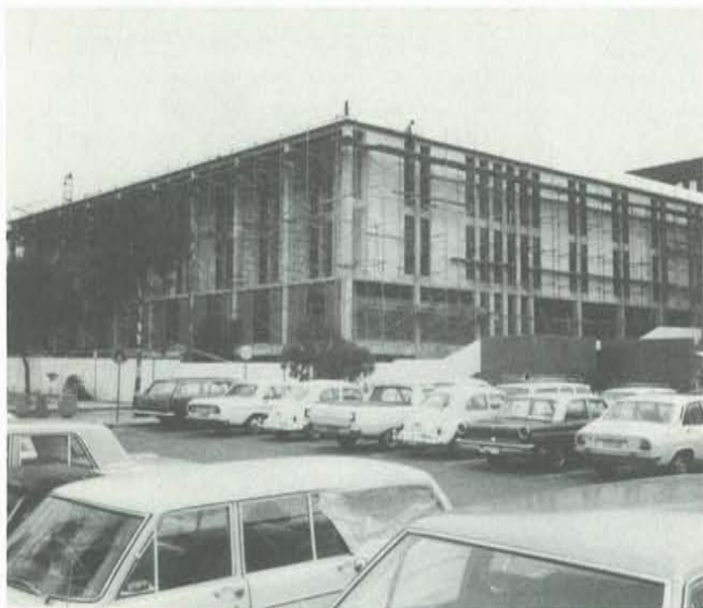
C.C.A.E. Building No. 1
