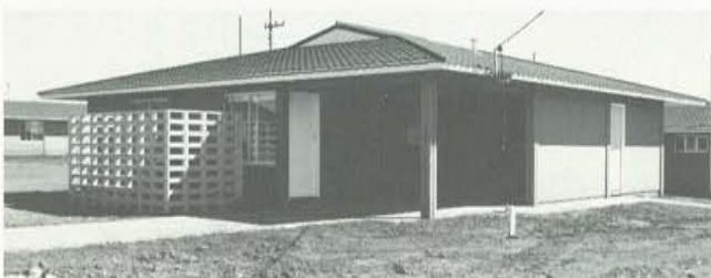
A completed pre-cast concrete home at Newman.
